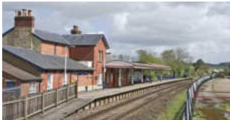
Figure 17 - The Railway Station and Station Works
