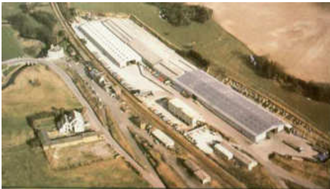
Figure 12 - Station Works in 1985
