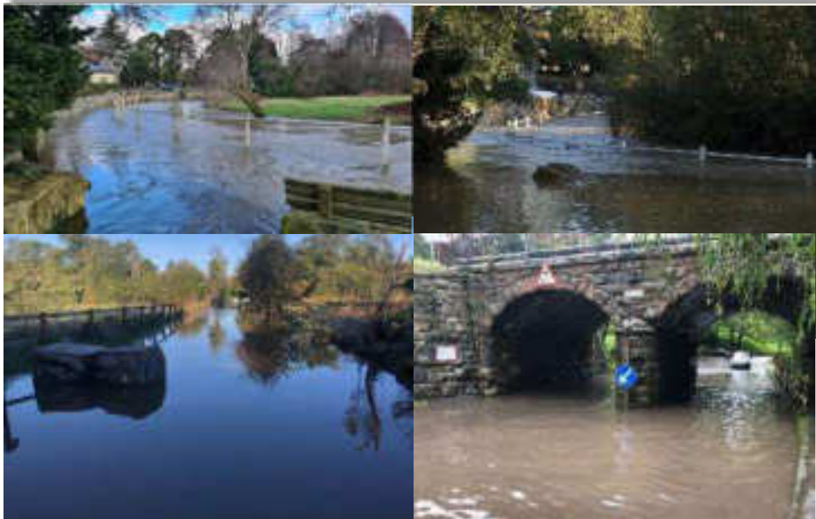
Figure 1 - Recent Flood Events affecting Stubbles Path and the Three Arch Bridge Pictures clockwise from top left, 16 th January, 2023, 20 th October, 2021, 2 nd November 2023 and 21 st October 2021
