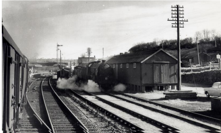
Figure 16 - Station Works in 1961
