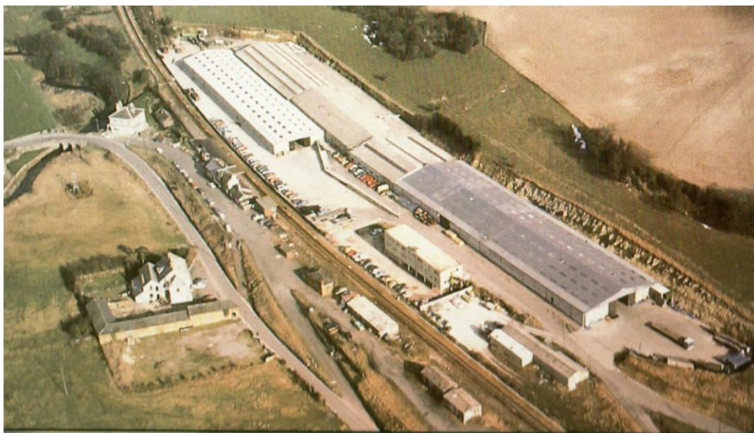
Figure 12 - Station Works in 1985
