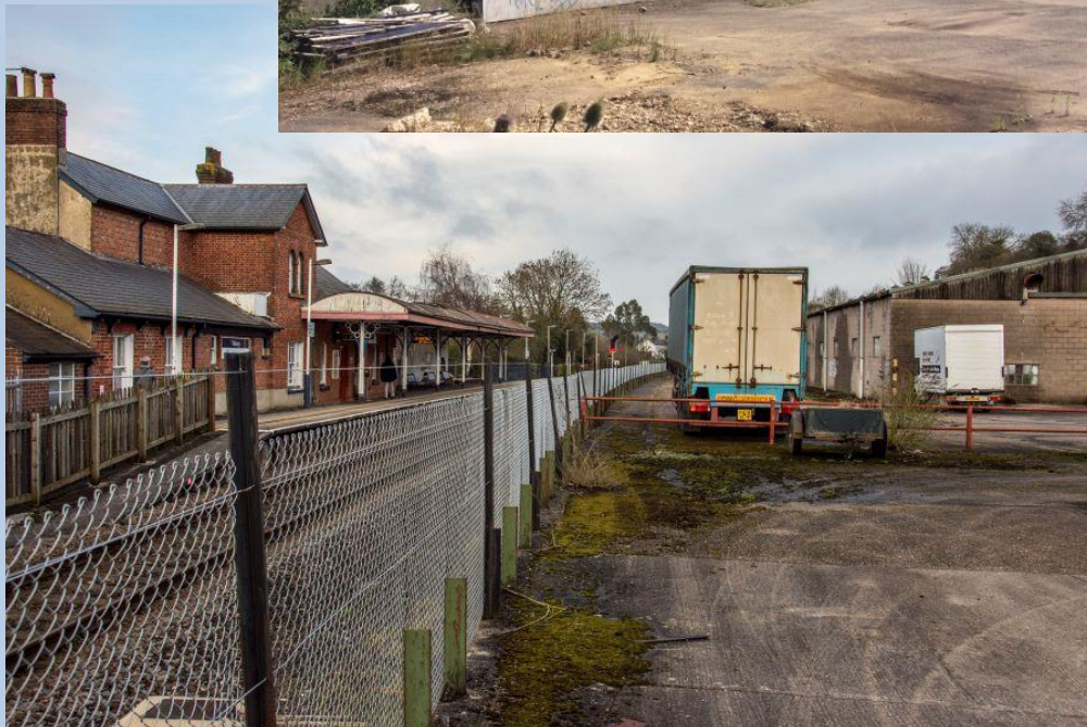
Above: part of the Boundary Transition Zone needing sensitive treatment, showing the Station Works site to the right of the railway station on the left.
