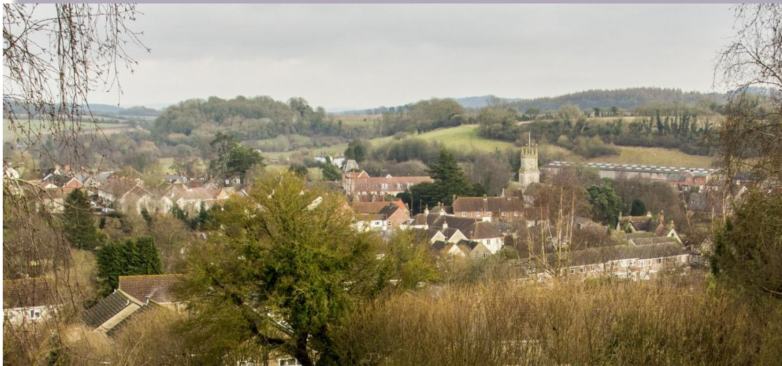
Figure 13 - Station Works Setting - View East from Mount Pleasant
