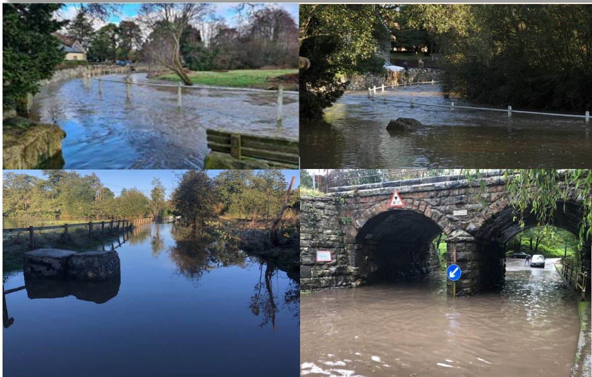
Figure 1 - Recent Flood Events affecting Stubbles Path and the Three Arch Bridge Pictures clockwise from top left, 16 th January, 2023, 20 th October, 2021, 2 nd November 2023 and 21 st October 2021
