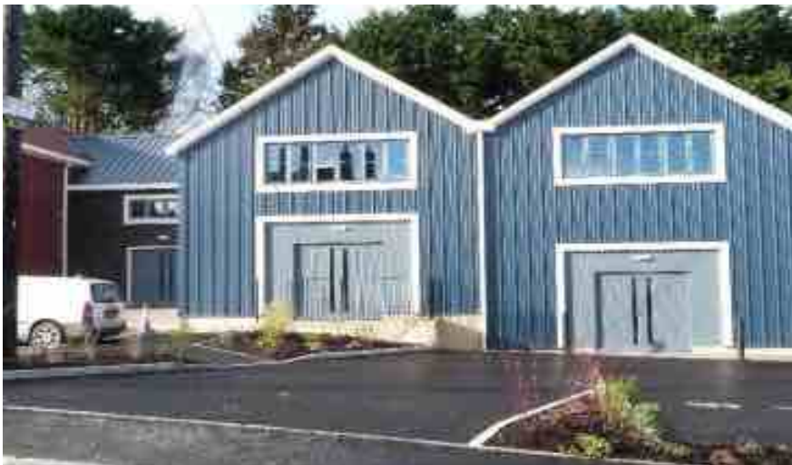
Figure 16 (above) - Commercial Units on the Wyndhams Estate, Hindon Lane
