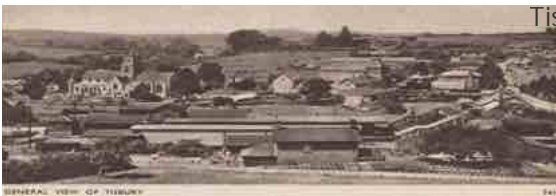
Figure 13 (left) Tisbury Railway Station, showing former Victorian bridge (late 19th Century).
