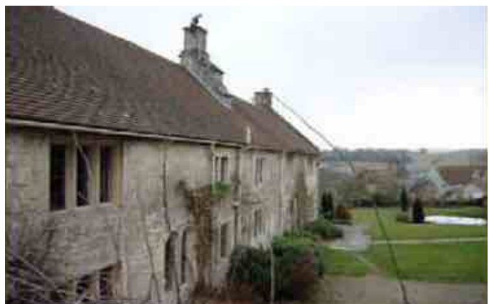
Figure 9 (above) Gaston Manor (Grade II* listed), High Street
