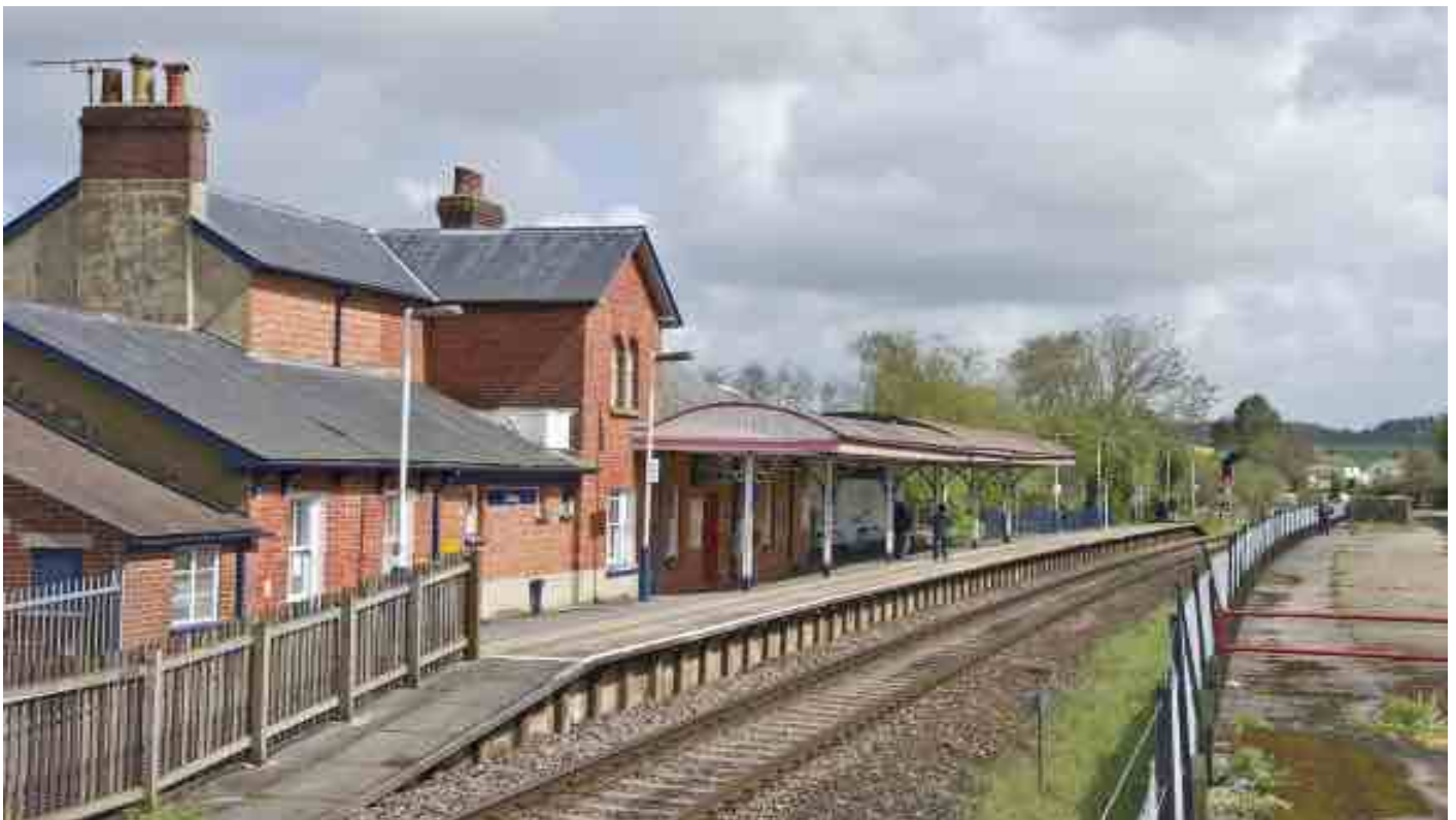
Figure 12 (above) Tisbury Railway Station, single track.
