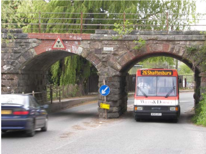
The Three Arch Bridge
