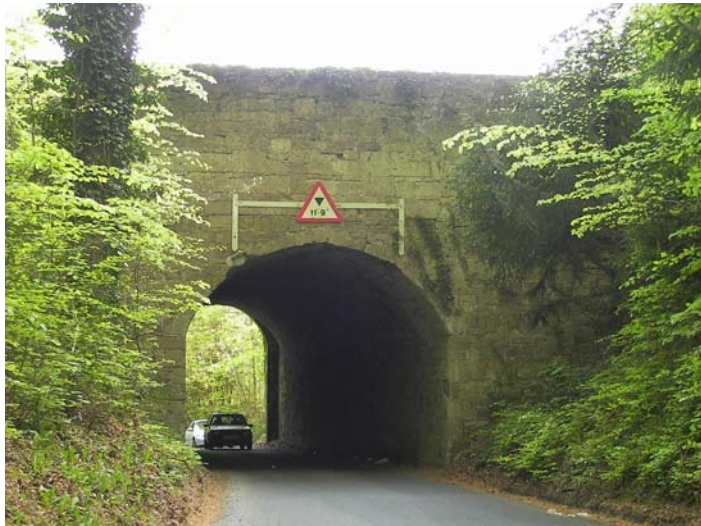
Hindon Road Tunnel
